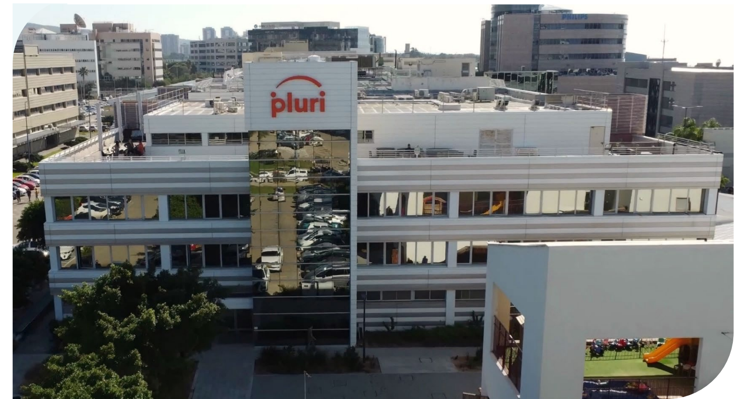
Flexible GMP manufacturing facility with excellent infrastructure
