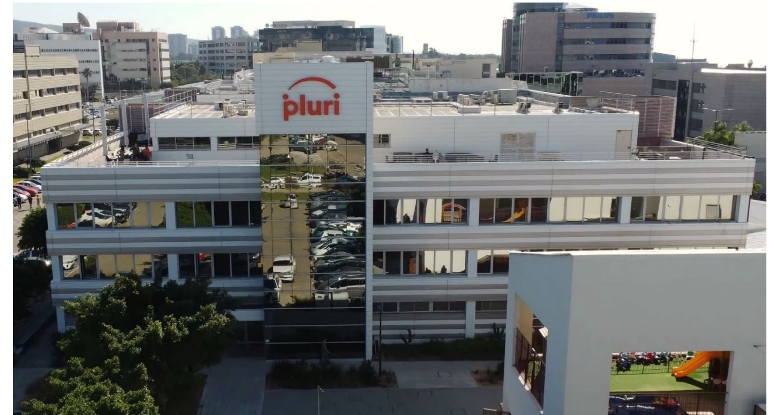
Flexible GMP manufacturing facility with excellent infrastructure
